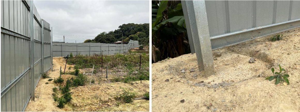
Photo Record for the Existing Fencing with openings at bottom surrounding the site
